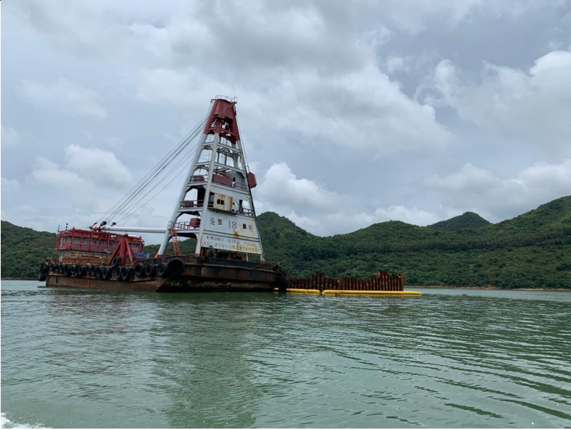
Silt curtain was deployed around the marine works area.
